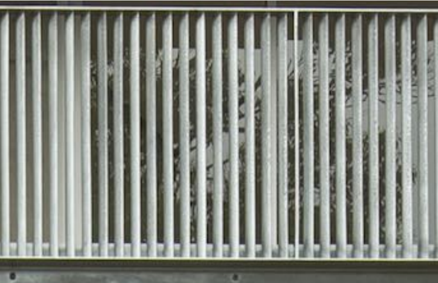
BAL 1 - Angled metal vertical members. Gal steel or aluminium
